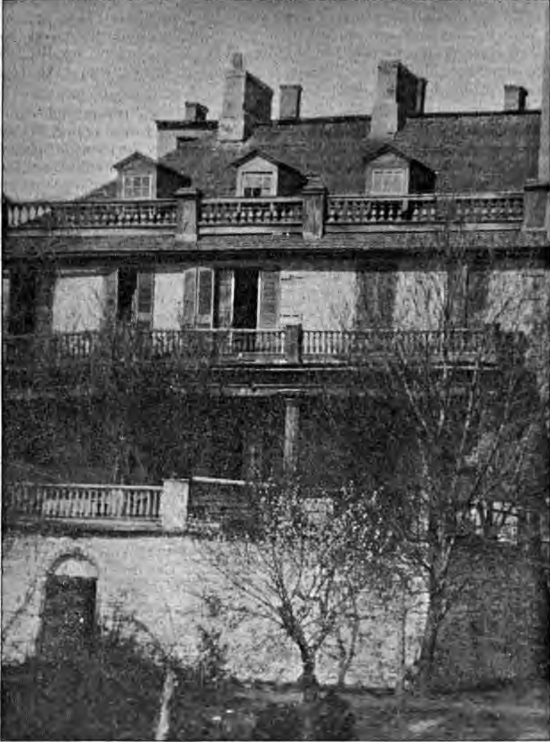
CARLYLE HOUSE, REAR VIEW.
